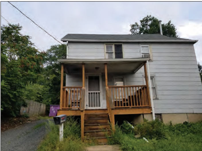
Figure 3: Front porch from River Road. Slight bend in porch roof and supports is visible.
