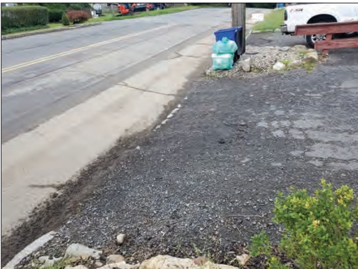
Figure 5: Deteriorated driveway and driveway apron leading to rear parking area.
