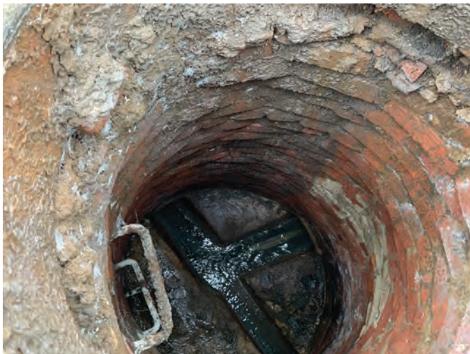
Image 19 - Manole # 5:: Brick arch line located at the intersection of River Road and Watchung Avenue.
