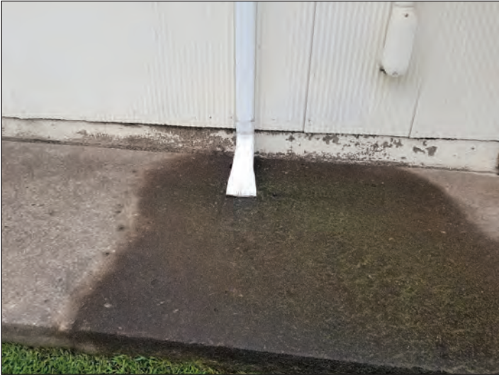
Figure 13: Damaged downspout shoe, with water soaking walkway below. Visible water damage to building wall.
