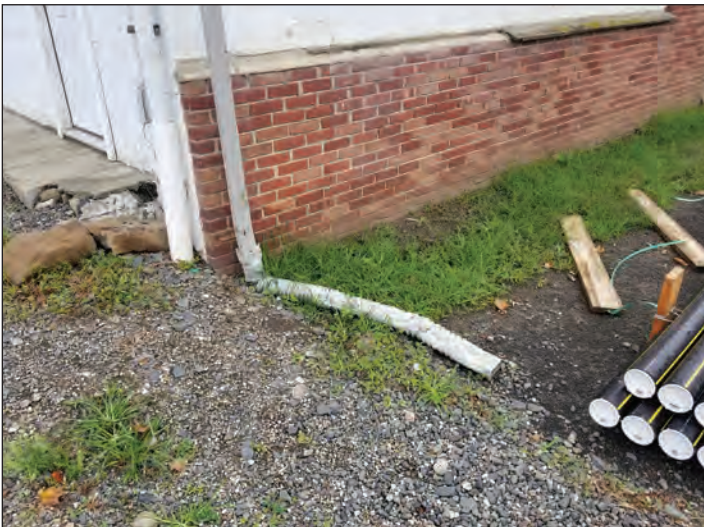
Figure 3: Downspout extender. Damaged walkway visible at building side. Missing masonry treatment on front facade.
