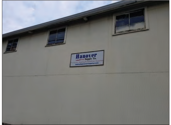
Figure 14: Faded paint and possible rotting of second story window frames.
