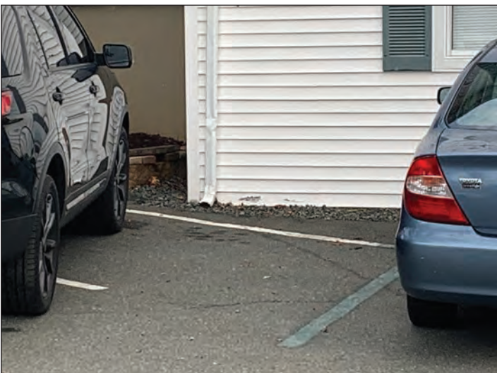
Figure 5: Downspout opening onto parking area near building wall.
