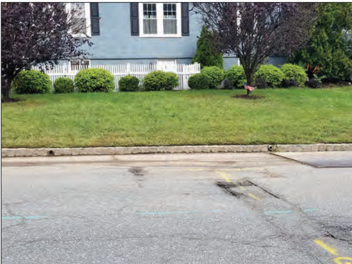
Figure 3: Stormwater outlets releasing into River Road cartway.
