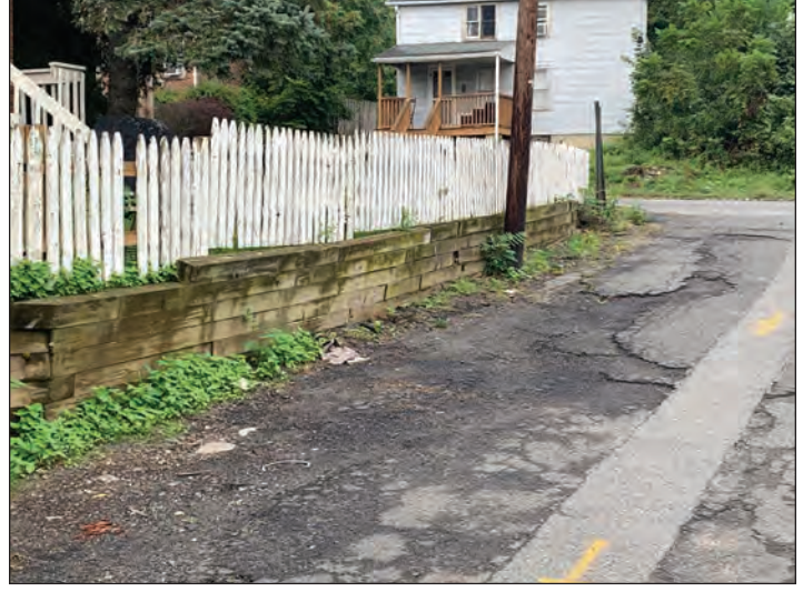
Figure 3: Deteriorated conditions on St. James Street, warped fence and retaining structures.
