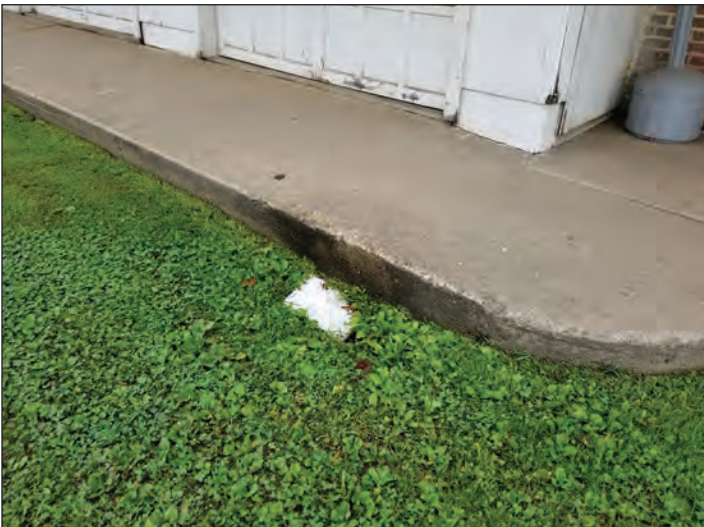
Figure 9: Marble block covering hole or ditch adjacent to walkway. Rotting siding visible on building.
