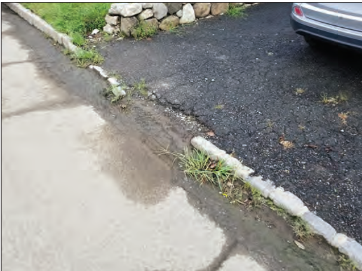
Figure 3: Damaged driveway apron and missing curb blocks.
