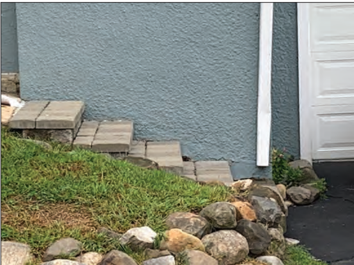
Figure 3: Downspout releasing onto steps, creating possibly slippery conditions during freezing weather.
