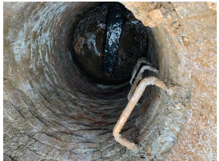
Image 6 - Manhole #2: Brick arch line located on River Road.
