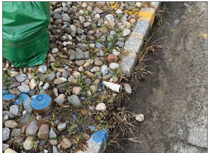
Figure 4: Damaged stormwater pipe opening into cartway. Visible sediment accumulation along curb.
