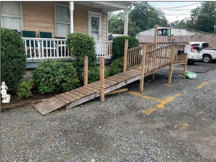
Figure 3: Unsafe wheelchair ramp with missing and failing rails.
