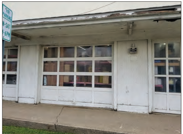
Figure 12: Rotting wood on eaves. Cracked walkway.
