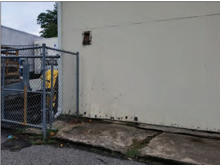
Figure 15: Rotting and warping of siding, deteriorated walkway.
