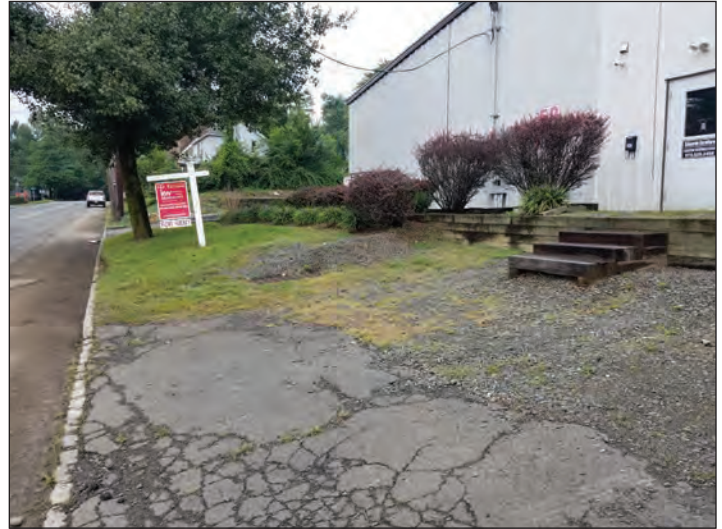
Figure 2: Steps to front entrance from deteriorated, inclining parking area.
