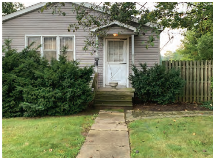
Figure 1: River Road building entrance. Incomplete railing system.
