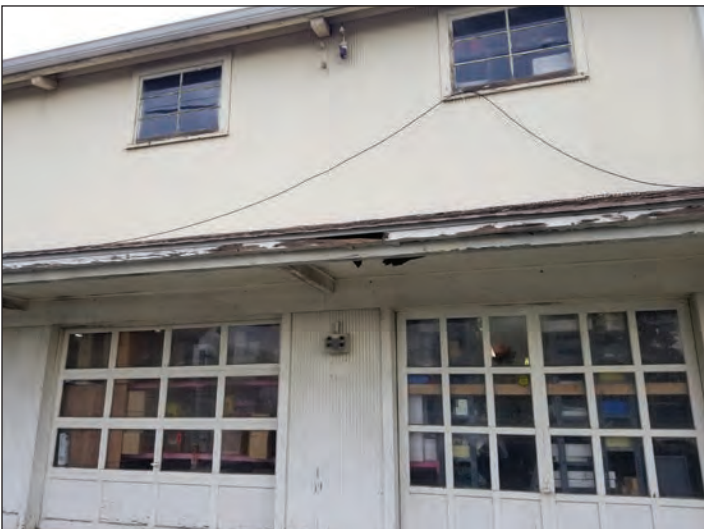
Figure 11: Rotting wood on eaves.
