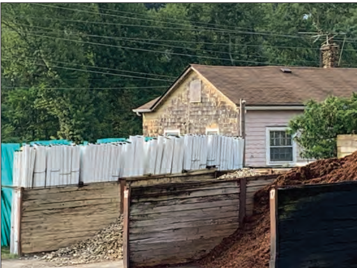
Figure 5: Rear of building visible from River Road. Deteriorated wood siding and bowing roof visible.
