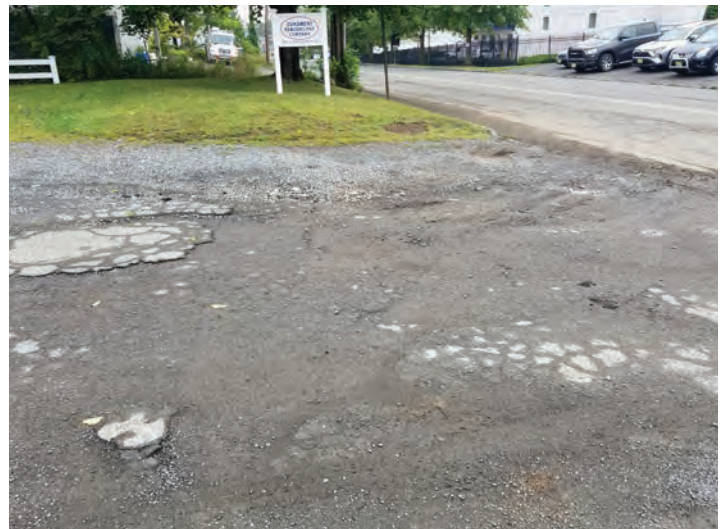
Figure 7: Driveway deterioration.
