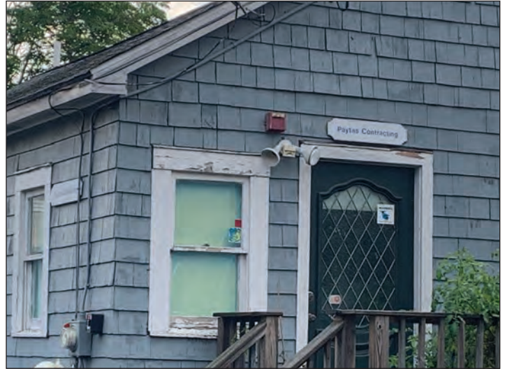
Figure 2: Rotting door and window frames. Moss accumulating on roof. Visible wear and shifting of siding materials.
