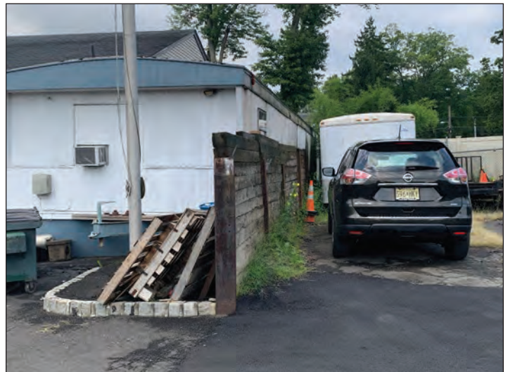
Figure 7: Rear property wall. Top of wall beginning to warp.
