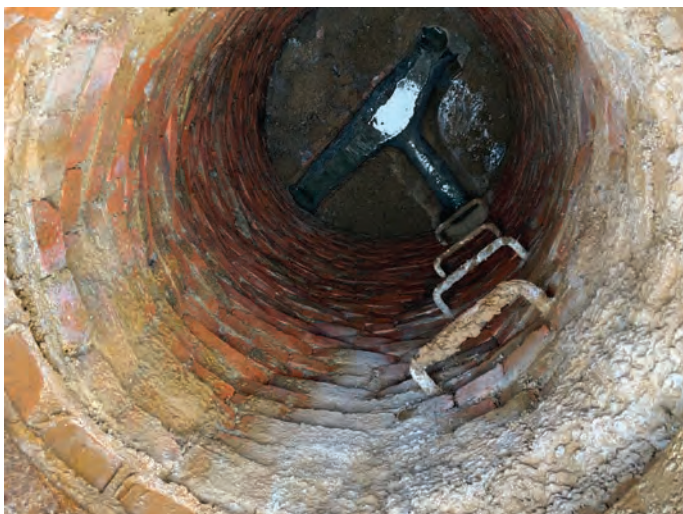
Image 13 - Manhole #4: Brick arch sewer line located on River Road.
