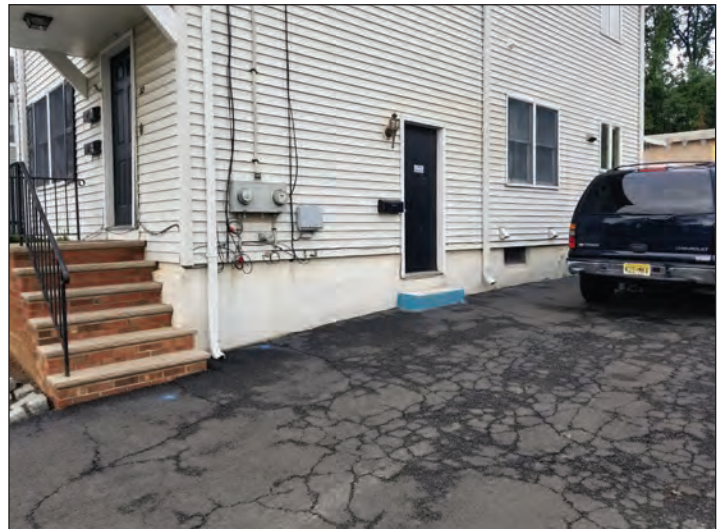
Figure 4: Side building entrance. Roof leader downspouts opening onto driveway near building wall and stairs.
