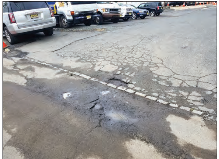
Figure 4: Damage to driveway entrance and cartway.
