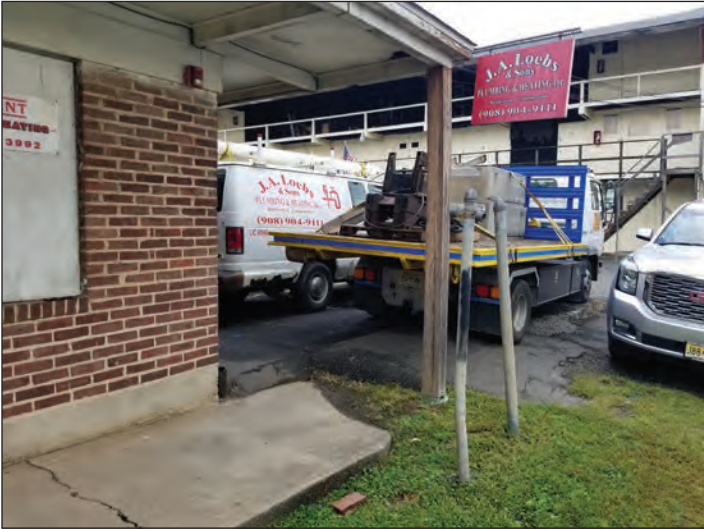
Figure 7: Cars parked adjacent to store. Lack of ADA accessibility due to abrupt grade change and overgrown pavement.
