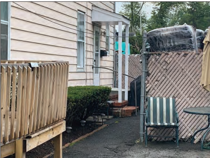
Figure 5: Steps to side building entrance (middle ground) and close up of failing ramp rails in lower left corner of image.
