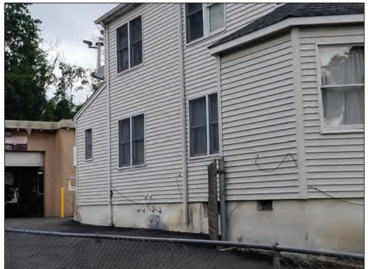
Figure 6: Side building wall. Roof leader downspouts opening onto driveway near building wall.
