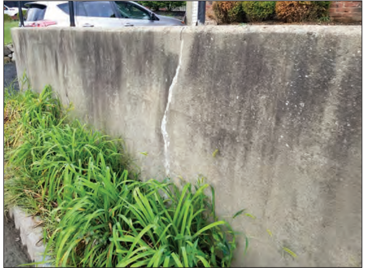
Figure 2: Patched crack in retaining wall along River Road.
