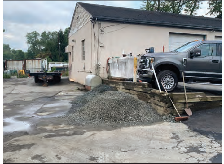
Figure 2: Gravel pile in front of collapsing retaining wall. Outdoor oil tank and other exterior equipment.
