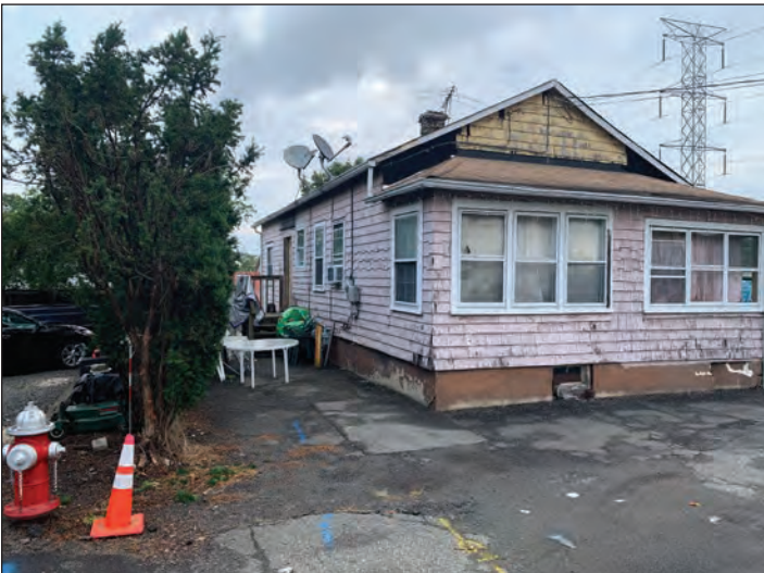
Figure 3: Other view of building with additional rotting wood features, damaged foundation.
