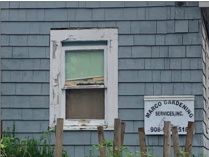
Figure 3: Rotting and damaged window.
