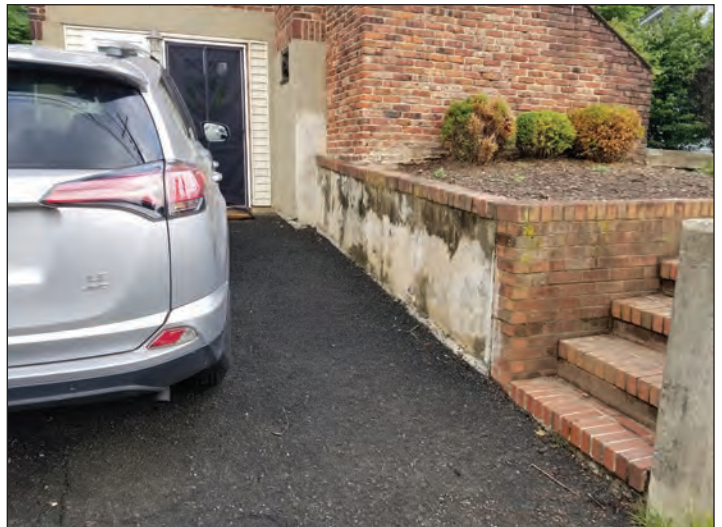
Figure 4: Water staining on retaining wall adjacent to parking lot.
