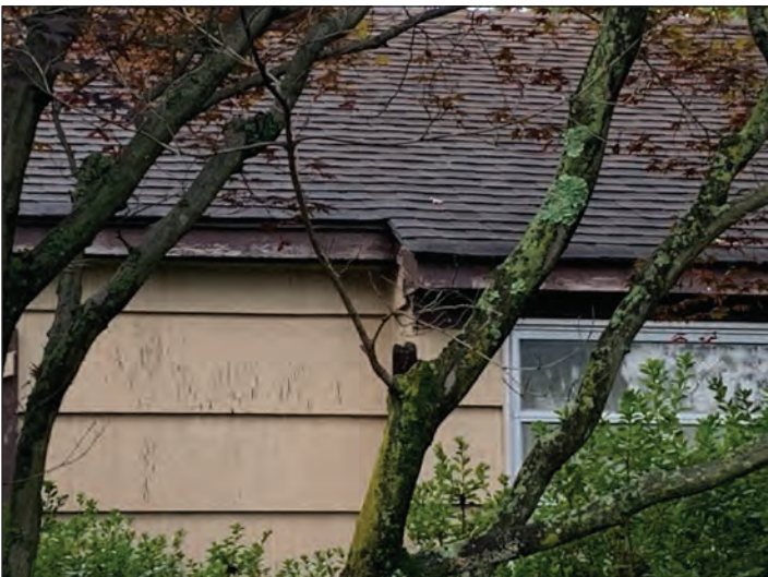
Figure 5: Faded paint and possible wood rotting on roof eaves and siding.
