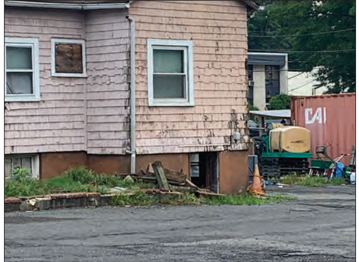
Figure 2: Open wall penetration, closer view of rotting siding, damaged curbs, downspout disconnected from gutter.
