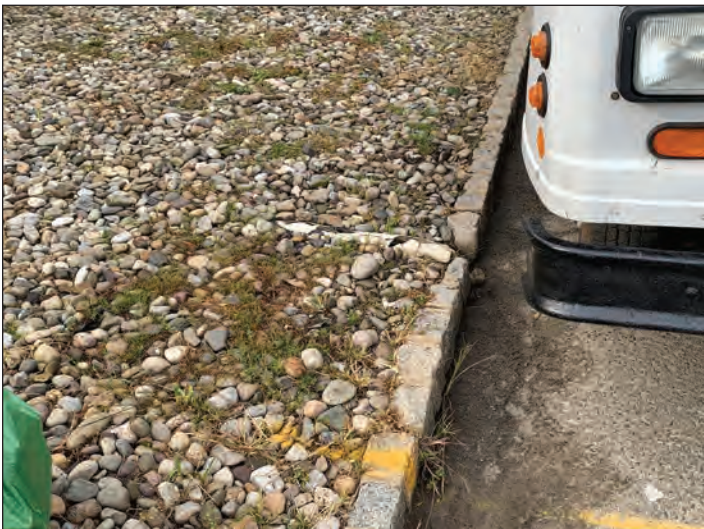
Figure 3: Damaged stormwater pipe opening into cartway. Visible sediment accumulation along curb.
