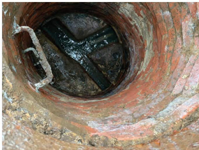
Image 18 - Manhole #5: Brick arch line located at the intersection of River Road and Watchung Avenue.
