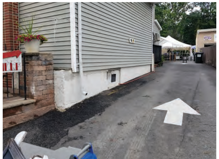
Figure 7: Downspout opening onto driveway near building wall. Visibly wet pavement surface area.
