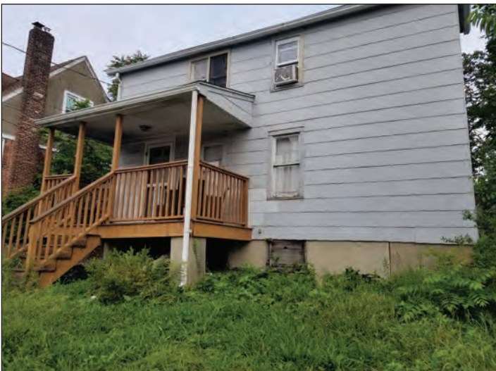
Figure 5: Northeast corner of dwelling. Slight rotting of wood window treatments.
