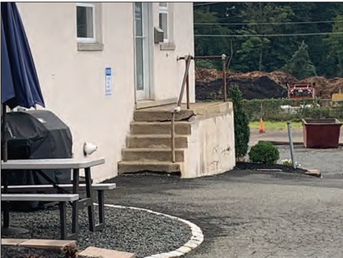
Figure 3: Deteriorated side door stairs, with missing safety rail.
