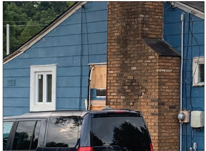
Figure 4: Another view of boarded-up windows/penetrations. Possible rotting wood on roof rake and window frames.
