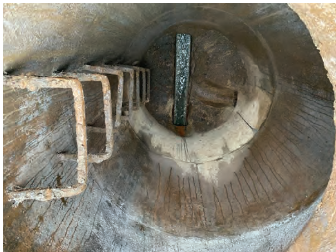
Image 7 - Manhole #3: Concrete sewer line located between two brick arch lines located on River Road.
