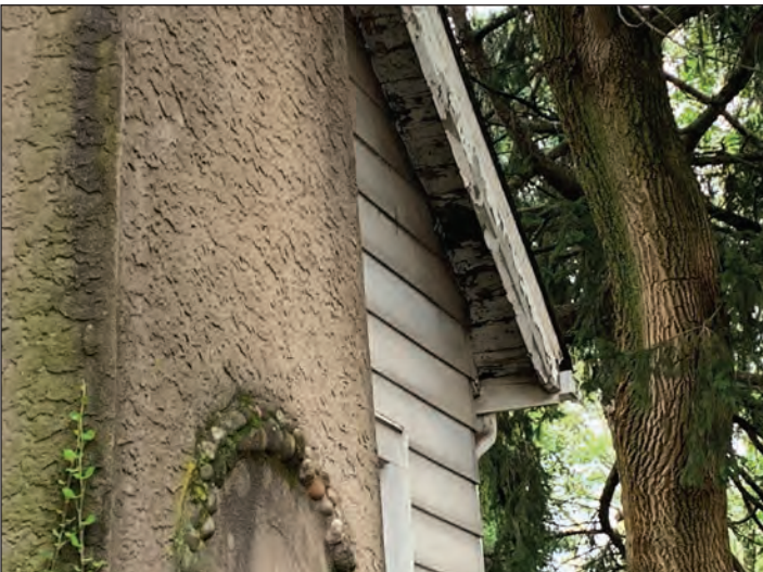
Figure 3: Faded paint and potentially rotting wood on dwelling eaves and siding.
