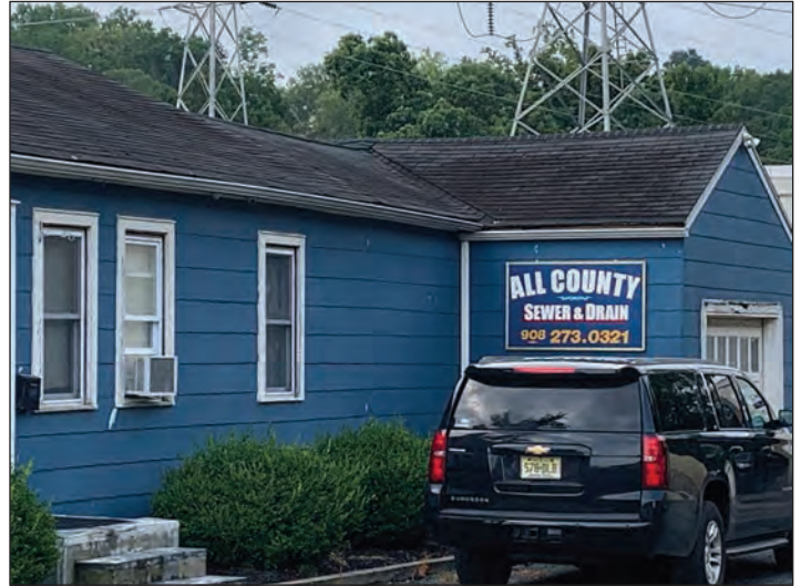
Figure 2: Close-up of building. Mild paint and siding wear, possibly indicative of rotting wood.
