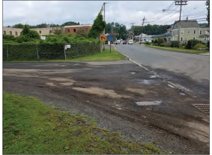
Figure 2: Driveway apron comprised of gravel and deteriorated pavement. Potholes forming.
