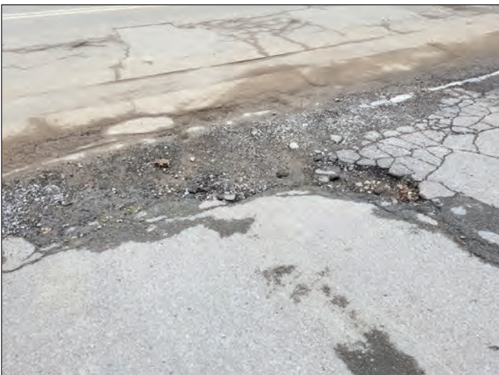
Figure 4: Damaged driveway apron on Lot 6.
