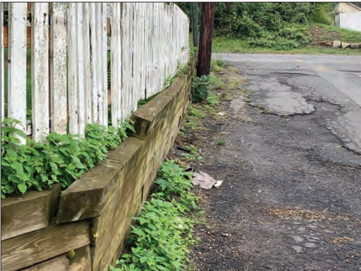
Figure 4: Close-up of displaced retaining structures. Mild wood rotting visible on fence.
