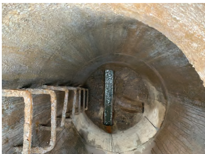
Image 9 - Manhole #3: Concrete sewer line located between two brick arch lines located on River Road.
