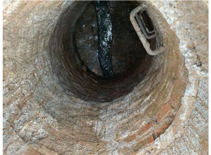
Image 2 - Manhole #1: Brick arch sewer line located on River Road.
