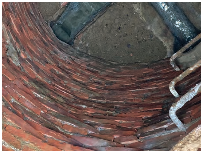
Image 14 - Manhole #4: Brick arch line located on River Road.
