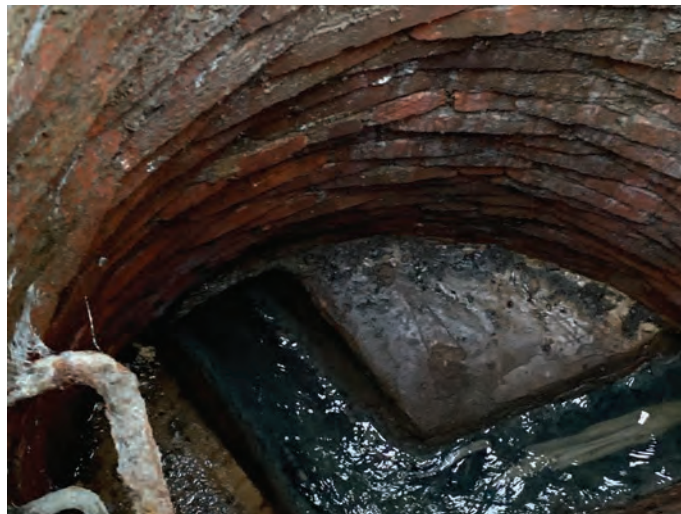
Image 20- Manole # 5:: Brick arch line located at the intersection of River Road and Watchung Avenue.
