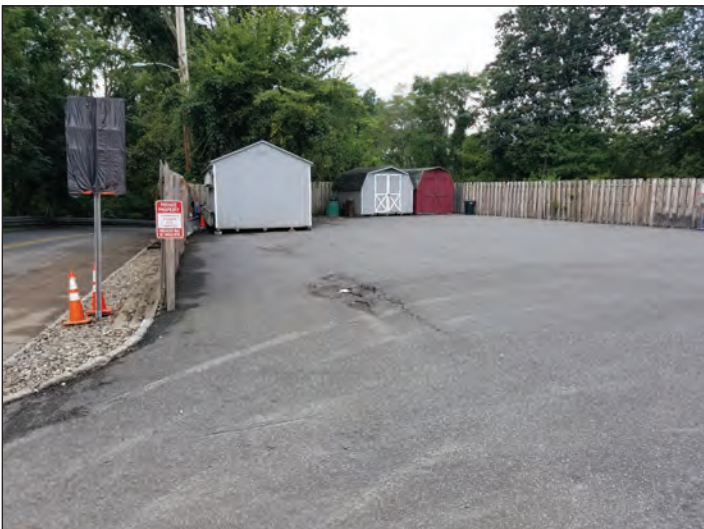
Figure 5: Storage sheds at rear of parking lot. Visible holes and depressions in parking surface.
