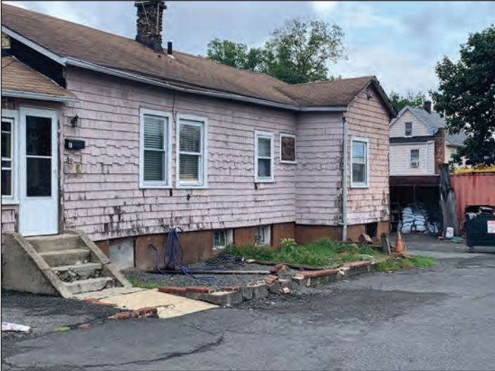
Figure 1: Office building with rotting siding, deteriorated chimney, collapsing gutters, plywood-covered windows, and unsafe stairs.
