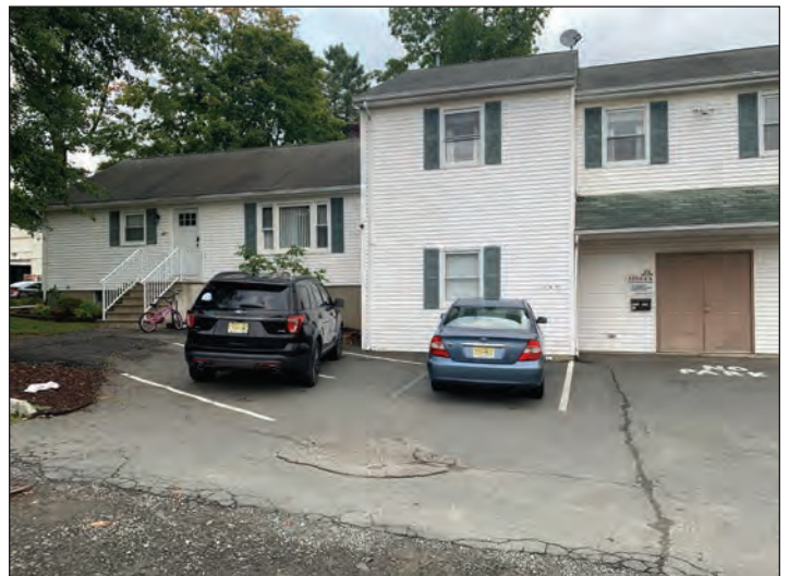
Figure 4: Inconsistent and unclear parking area striping, including a nonconforming ADA parking space.
