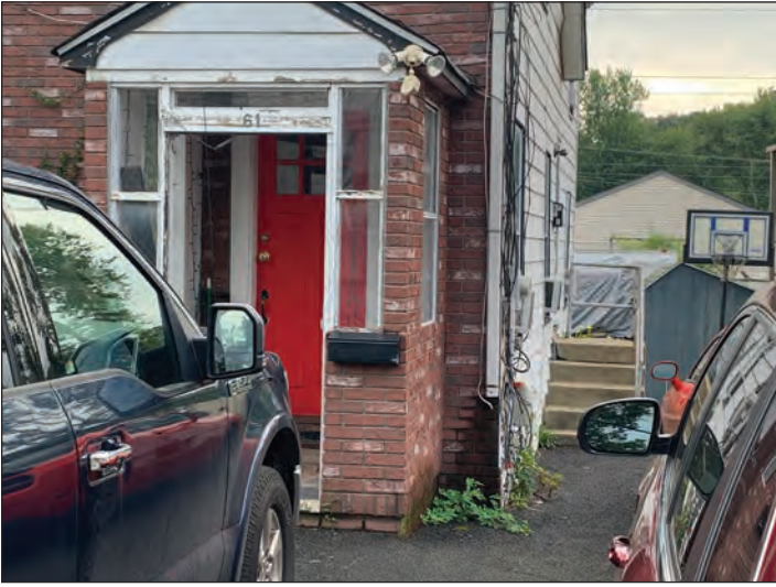
Figure 2: Downspout opening onto building wall, which is visibly wet from a recent storm.
