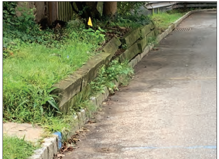
Figure 4: Collapsing and displaced wood railroad ties with retaining wall function.
