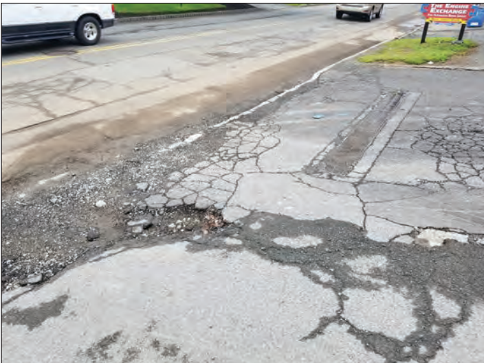
Figure 3: Deteriorated driveway to rear service shop.
