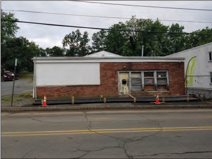
Figure 1: Front of building. Rotting wooden door, frames. Water stained brick. Outdoor storage in front yard.
