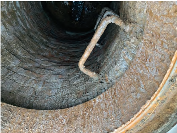
Image 5 - Manhole #2: Brick arch line located on River Road.
