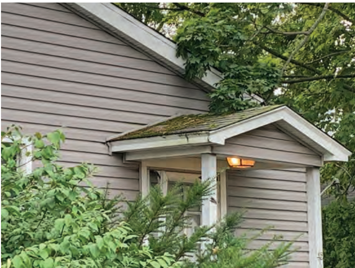
Figure 2: Moss and plant material accumulation on roof.
