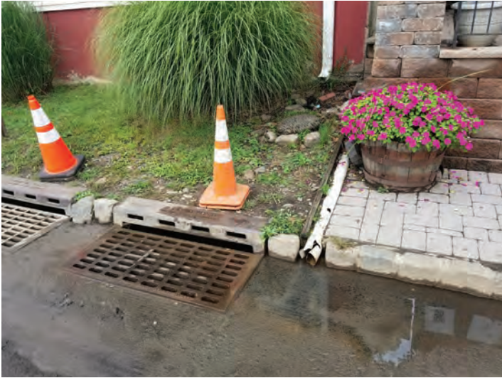
Figure 7: Stormwater collecting near drain in River Road cartway.
