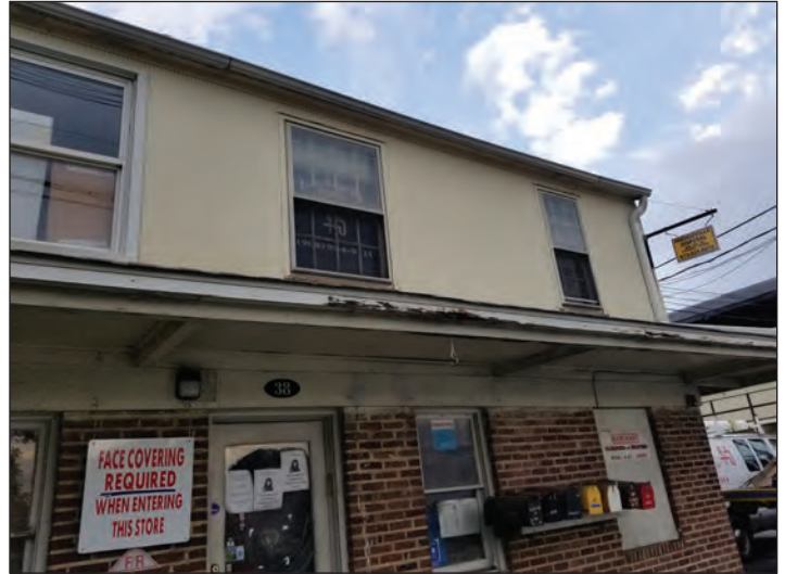
Figure 8: Rotting wood on eaves.
