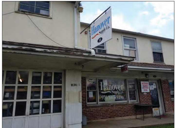
Figure 10: Rotting wood on eaves. Roof leader opening over walkway.
