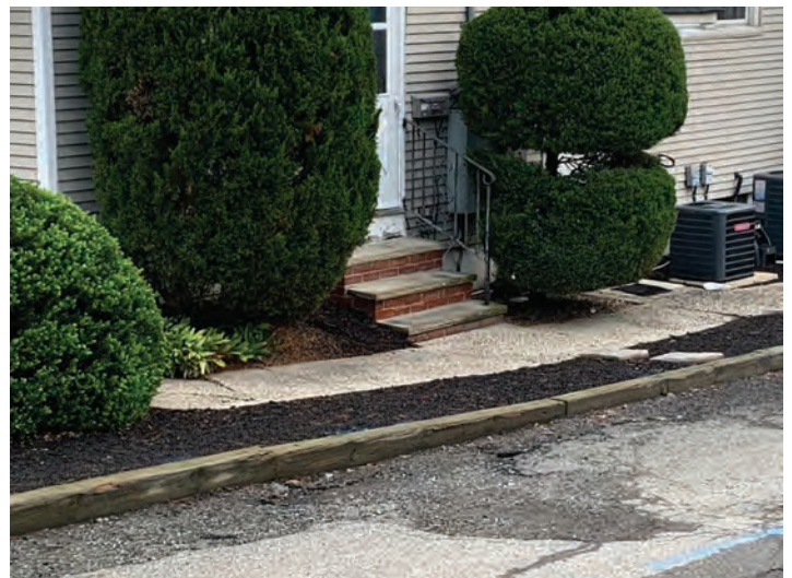
Figure 4: Steps to side entrance. Risers not equal heights. Only one handrail provided.
