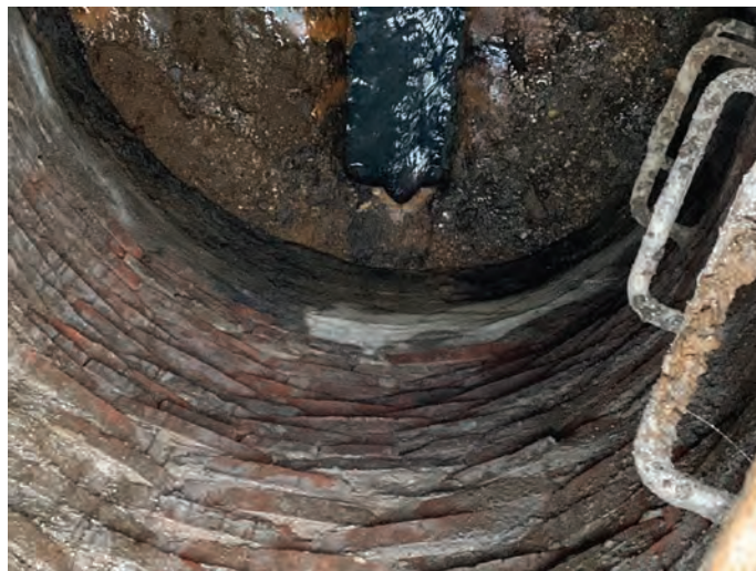
Image 12 - Manhole #4: Brick arch sewer line located on River Road.
