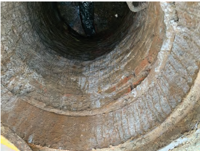
Image 3 - Manhole #1: Brick arch line located on River Road.
